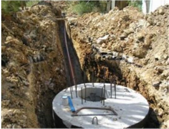
Manhole Construction and Pipe Laying
