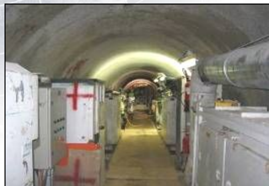
Hydraulic Tunnel Under Execution
