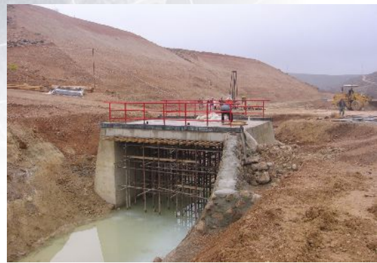
Construction Works - Package 1
