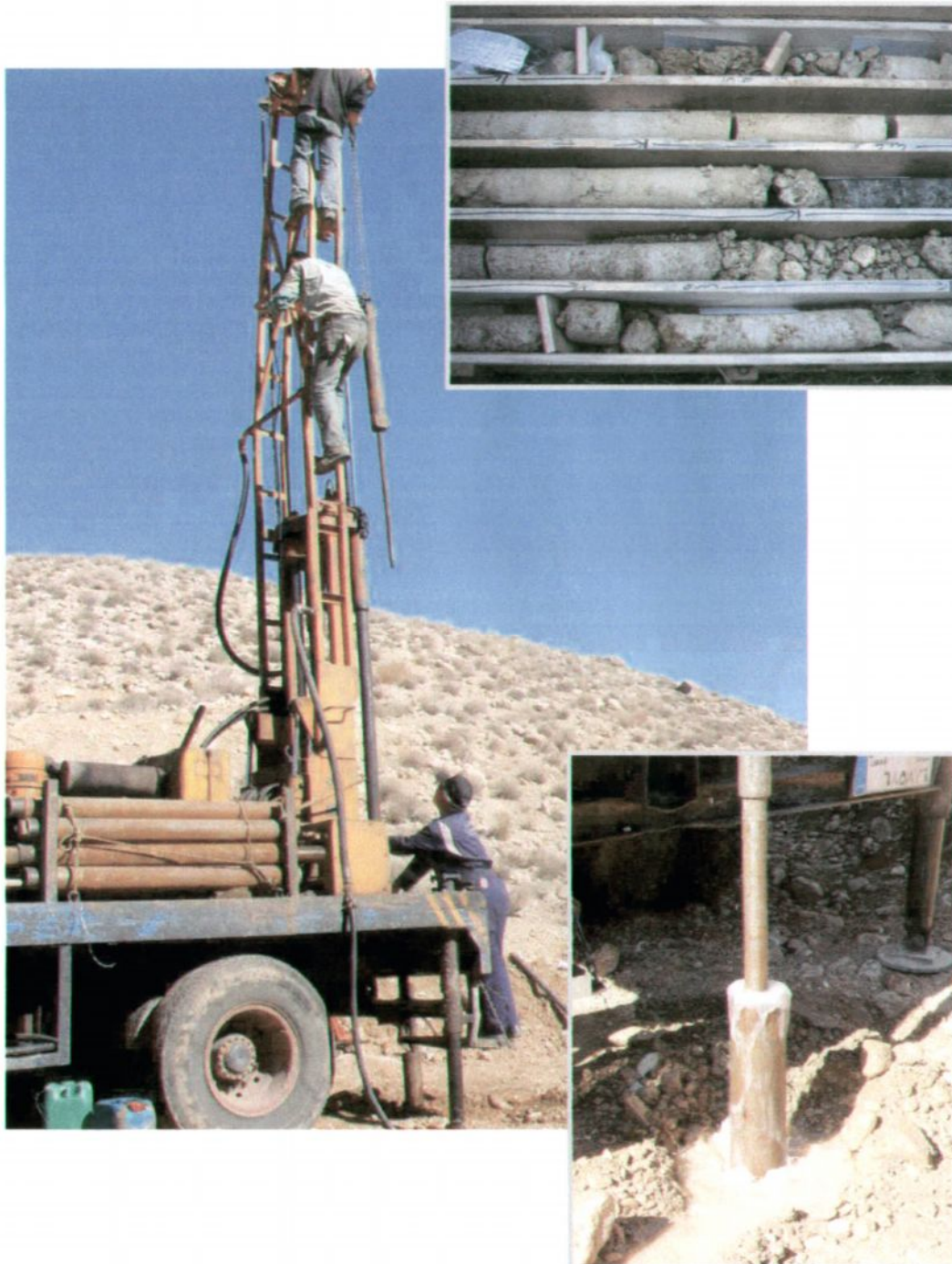
Geotechnical Investigation Works
