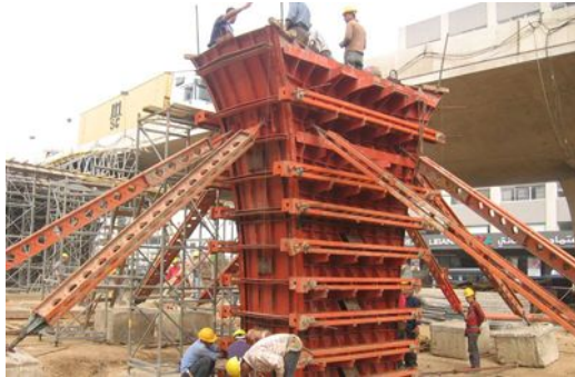
Dora Overpass - Formworks Works
