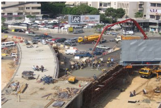
Hayek Overpass - Concrete Casting
