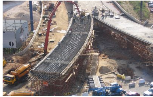
Hayek Overpass - Concrete Casting
