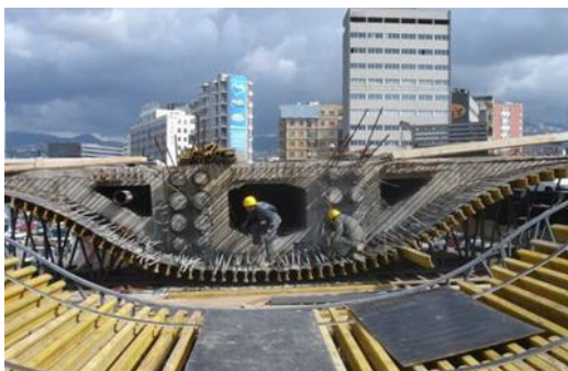
Dora Overpass - Formworks Works
