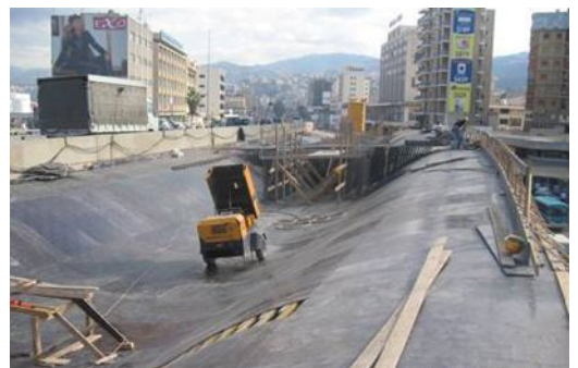
Dora Overpass - Formworks Works
