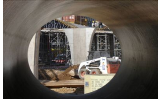
Scaffolds View Through Pipes
