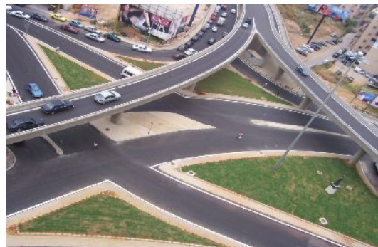
Hayek Overpass - Completed Works
