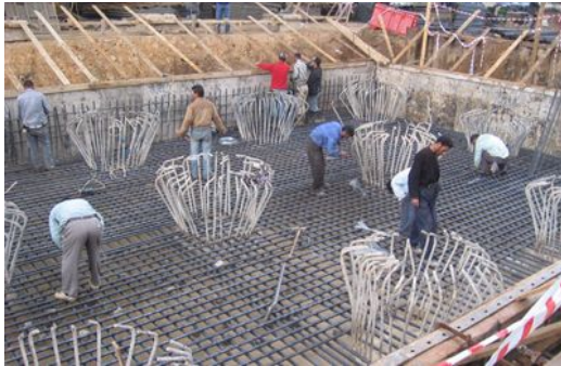
Dora Overpass - Reinforcement Works
